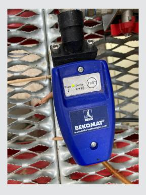
\*After running the condensate drain, please allow your compressors to again build pressure before testing functions. Also ensure the pressure is maintained without wash function use to prove the moisture drain is not leaking air.
