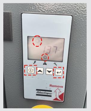
\*If your wash functions are currently not operational and you find your air compressors to be out of run mode, after setting your compressor to run mode, allow a few minutes for your compressors to build air pressure before testing wash functions.
