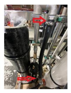
**5.** Remove the piping bracket and piping connected to Solenoid E.
