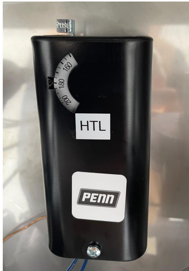
Figure 4 - P-HD-1010 – High Temp Limit Switch
