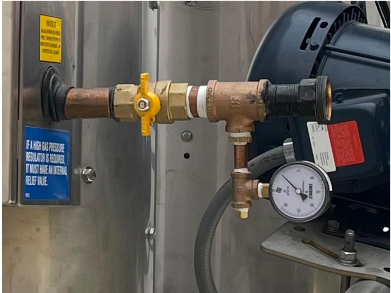
Figure 7 - External Gas Gauge Assy (P-HD-1021)
