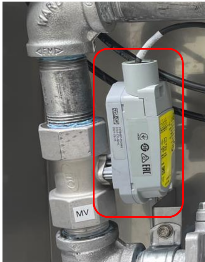
Figure 10 – Modulating Gas Actuator (P-HYD-2172)
