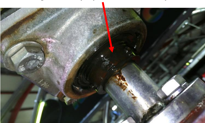
Sign of leaky hydraulic motor oily shaft
