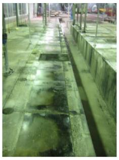
2. Remove floor and excavate according to Belt Pit Plan, leaving wash equipment in place.
