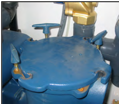
Basket Strainer with one dogear bolt removed and lid rotated for removal
