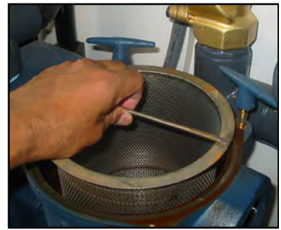
Basket Strainer being removed
