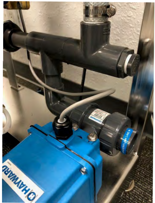
PW200/300/350 Underflow Plumbing (Front View)
